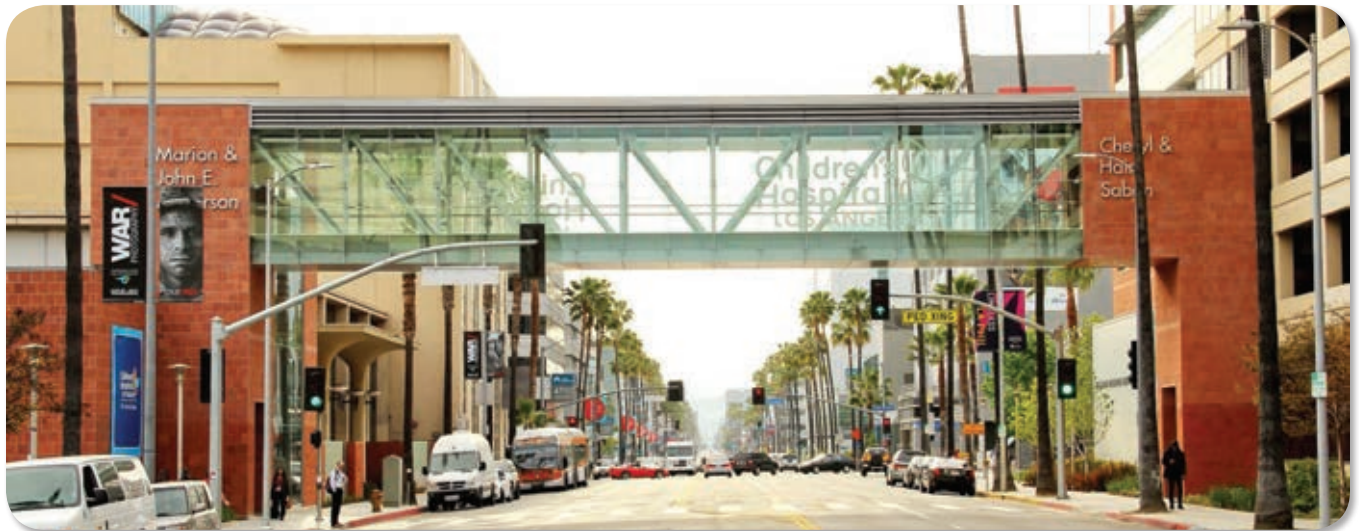
The new bridge over Sunset Boulevard connects wings of the CHLA campus
